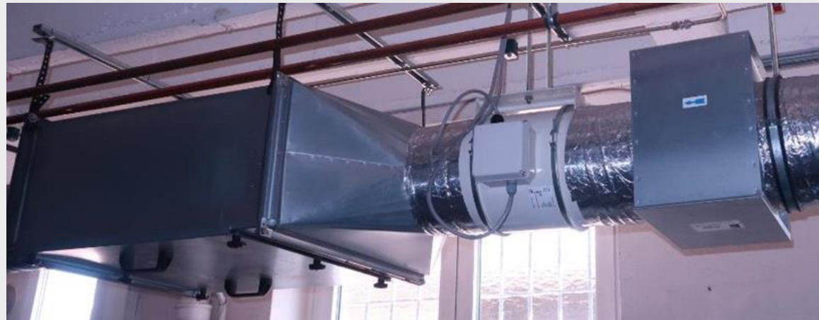
Fig. 12: Air fine filter, tube fan and air pre-filter of the exhaust air system
