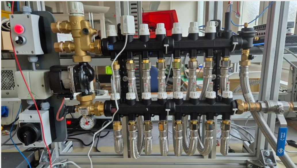
Fig.8: Application of the thermoelectric control valve FTV in the heating circuit manifold
