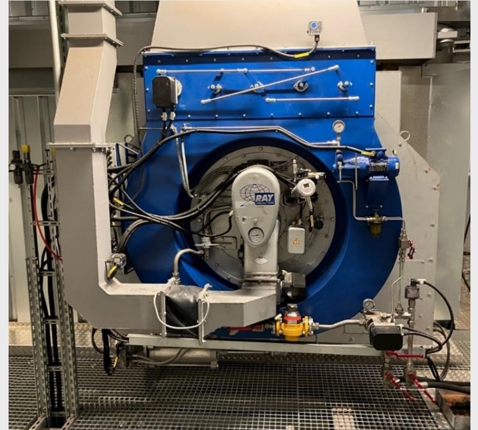
Fig.12: RAY Egelhof burner in the power station (RAY rotary burner BGE 25000)
