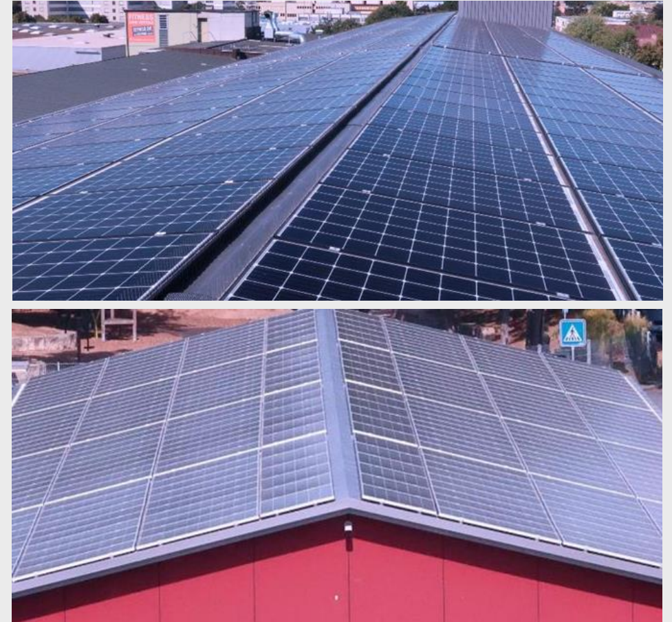
Fig. 10: Roof area of main and storage building in Fellbach
