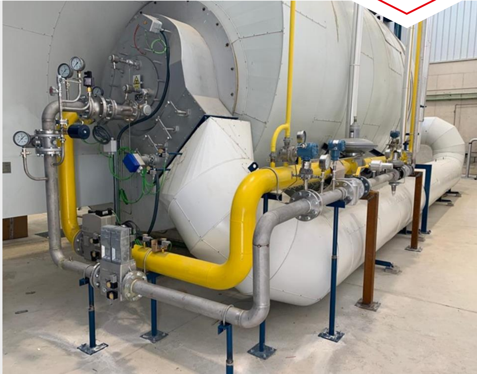
Fig. 6: RAY-EGELHOF Process heat from hydrogen with lowest nitrogen oxide emissions (Location: Cáseda, Spain)
